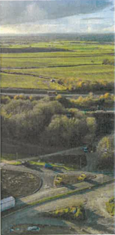
Following a rollercoaster ride through planning and financing, Amey's Allerton Waste Recovery Park is now up and running and will treat 50% of the household waste generated in the area by 2020.
