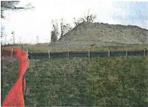
Stockpiled Excavation Material
