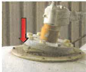
Leaking Gaskets
