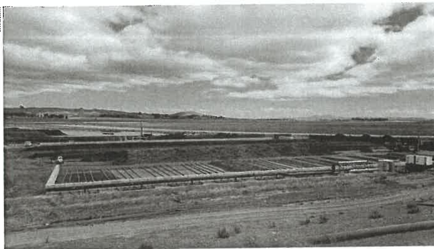
Optimizing airspace with mechanically stabilized earth berms
