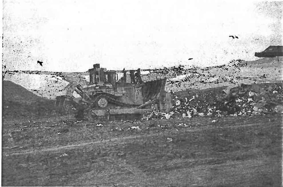
Dozer landfill work
