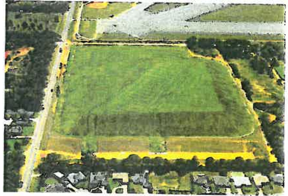
The 25-acre Saufley Field C&D landfill was capped using a "soiless" system.
