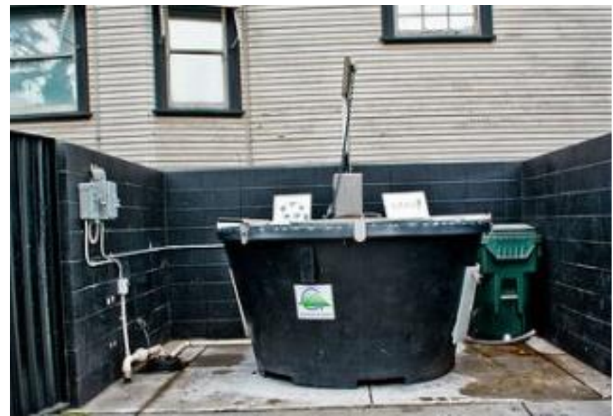
Earth Tub system behind LEED-certified Hot Italian Pizza and Panini Bar in downtown Sacramento
