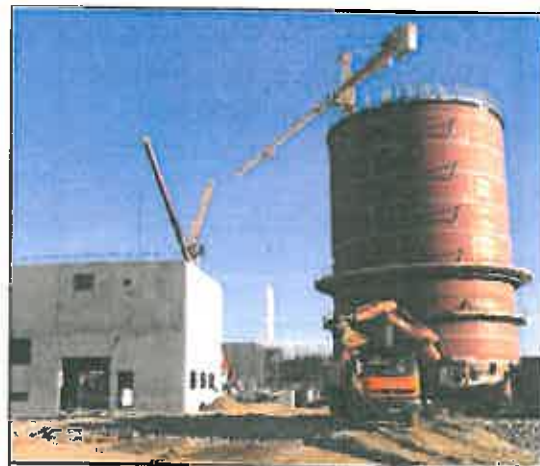
Credit: OWS A dry anaerobic digester under construction in Bourgen-Bresse, France
