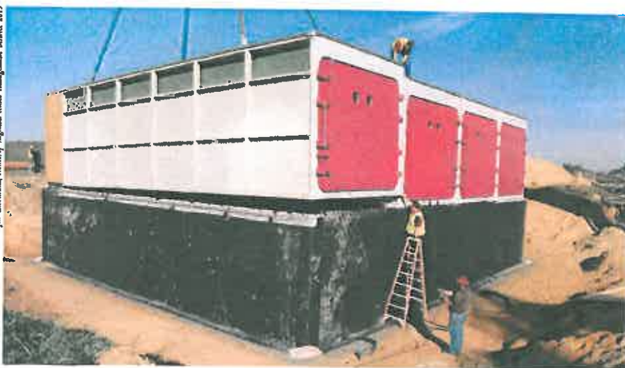
Exhibit 2. Last of four digesters installed in place
