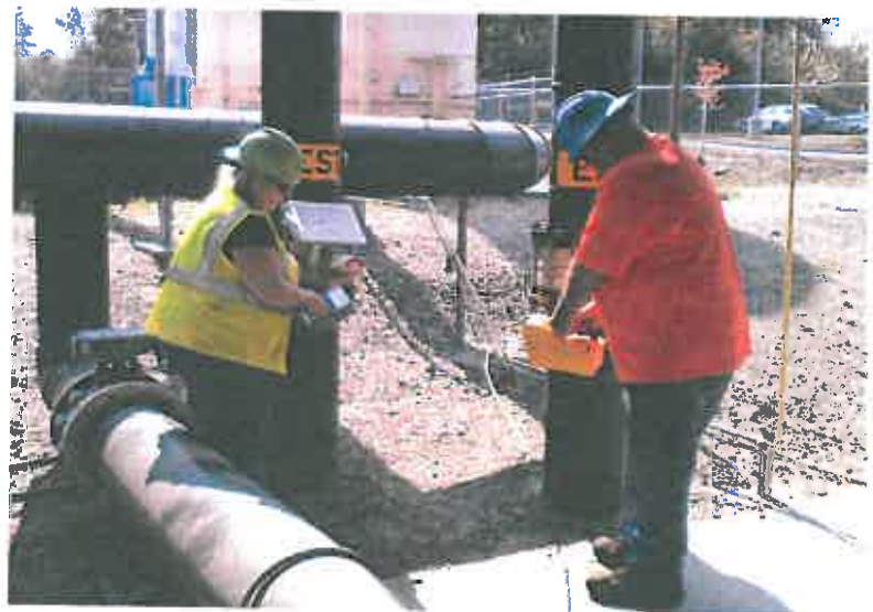
Workers check on methane levels at the Cathcart landfill in Snohomish County, Wash.
