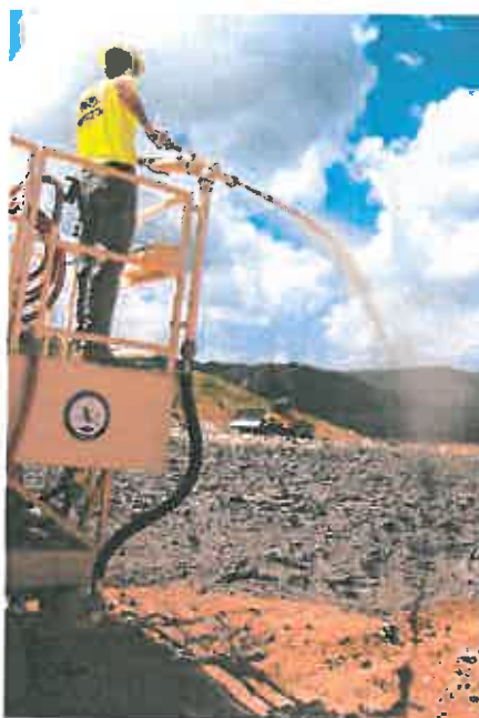
A Posi-Shell spraying
